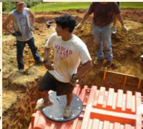
Matt and the team celebrate after successfully placing the holding tank for the septic system. Digging is done the old fashioned way because the worksites are located up in the mountains and it is difficult to get heavy machinery to dig the holes and trenches.
